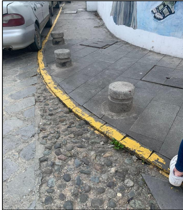
Curb Ramp in Luis Cordero Neighborhood
