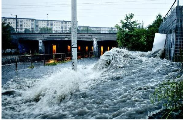
Figure 13 – Skybrud 2011 Flooding (Nielsen, 2011)
