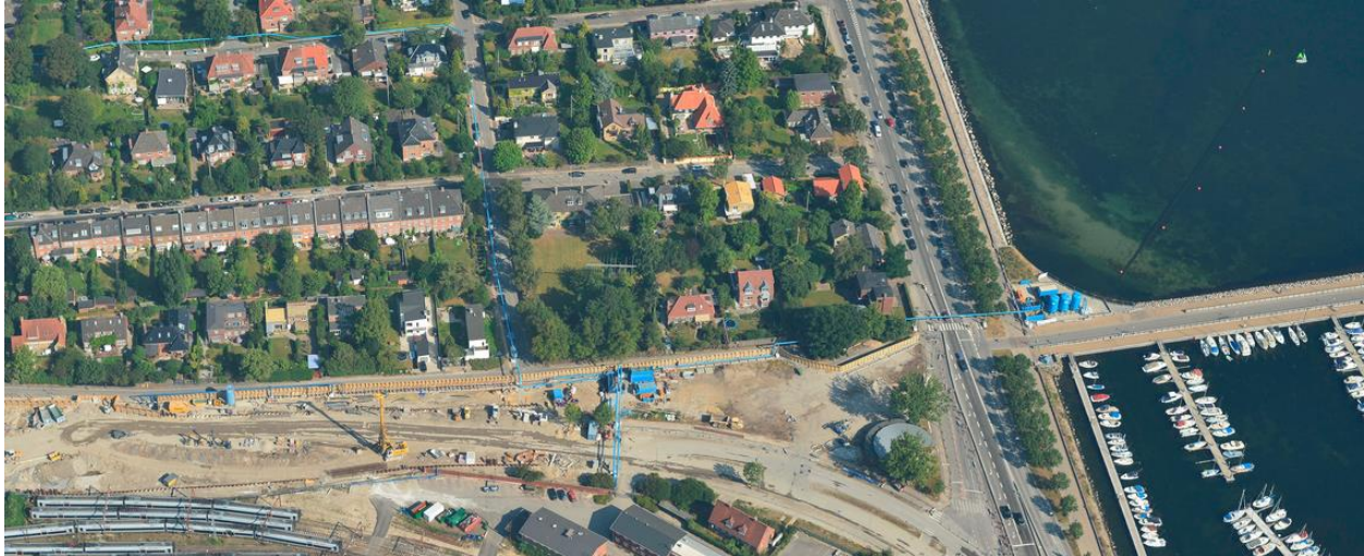
Figure 28 - A View of Strandvænget and the O2 from the South
