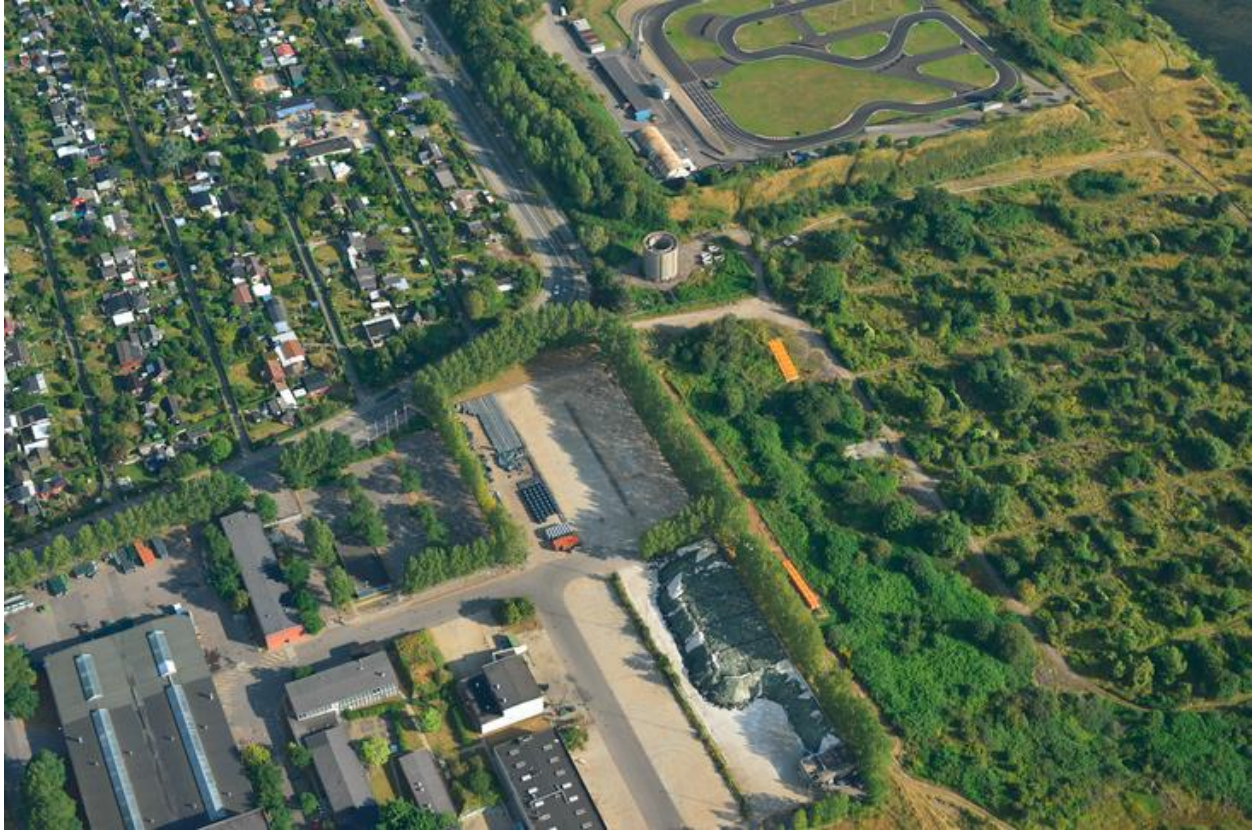
Figure 37 – Kløvermarksvej, View from the South
