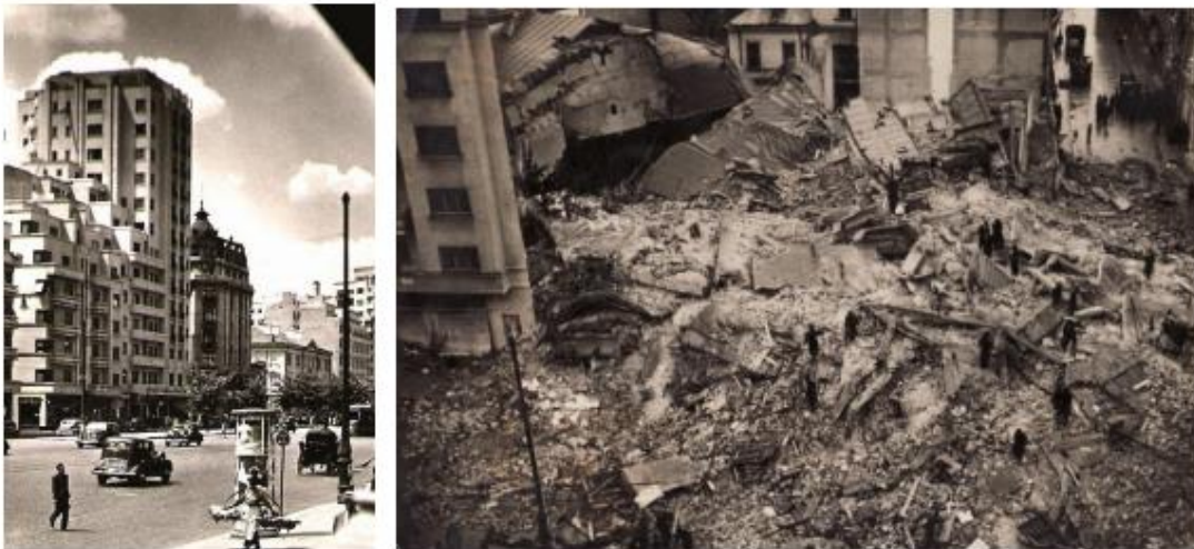
Figure 2.6: The Carlton Block before collapse (left) and after collapse (right). Georgescu, E & Pomonis, A (2012).
