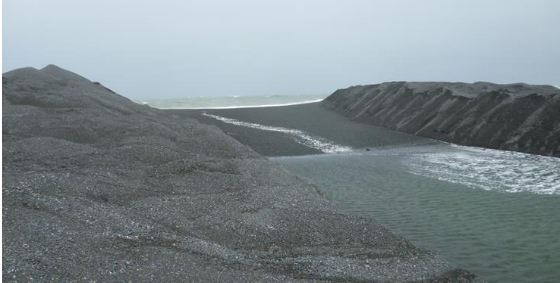
FIGURE 2.10 FAILED OPENING OF THE LAKE ONOKE SPIT, [PHOTOGRAPH GWRC, 2011]
