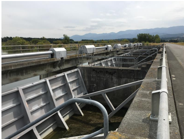
FIGURE 2.2 THE GEOFFREY BLUNDELL BARRAGE GATES
