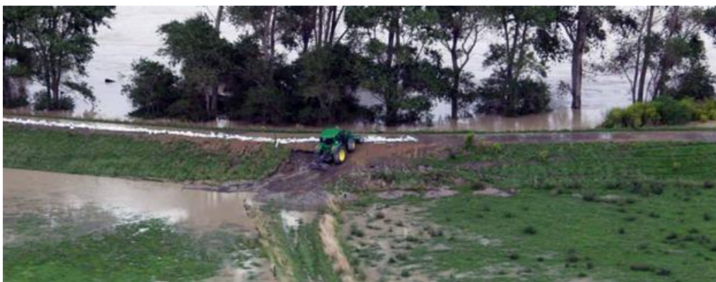
FIGURE 2.4 STOPBANKS ALONG THE RUAMAHANGA, [PHOTOGRAPH GWRC, N.D.]
