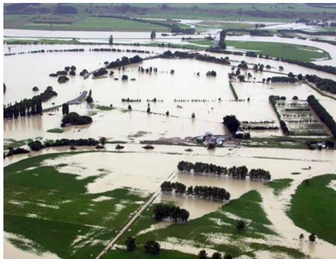
FIGURE 2.11 FLOODING OVER STATE HIGHWAY 53, MARTINBOROUGH, 2004. [PHOTOGRAPH GWRC, 2004]
