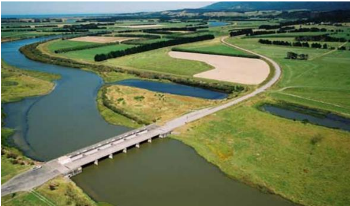
FIGURE 2: THE GEOFFREY BLUNDELL BARRAGE, [PHOTOGRAPHS GWRC, N.D.]
