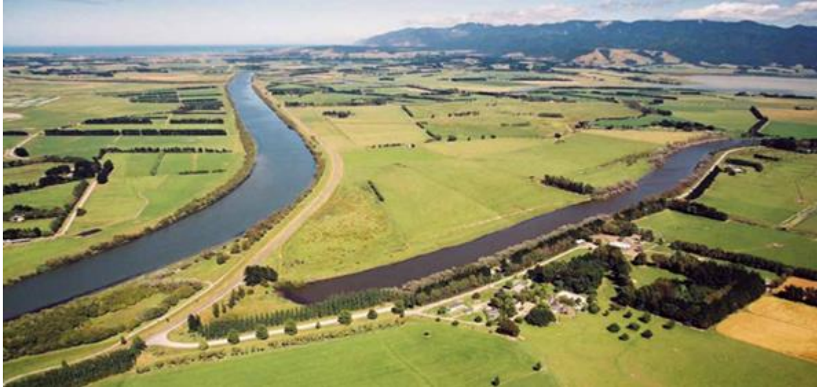
FIGURE 4: RUAMAHANGA RIVER DIVERSION, [PHOTOGRAPH GWRC, N.D.]
