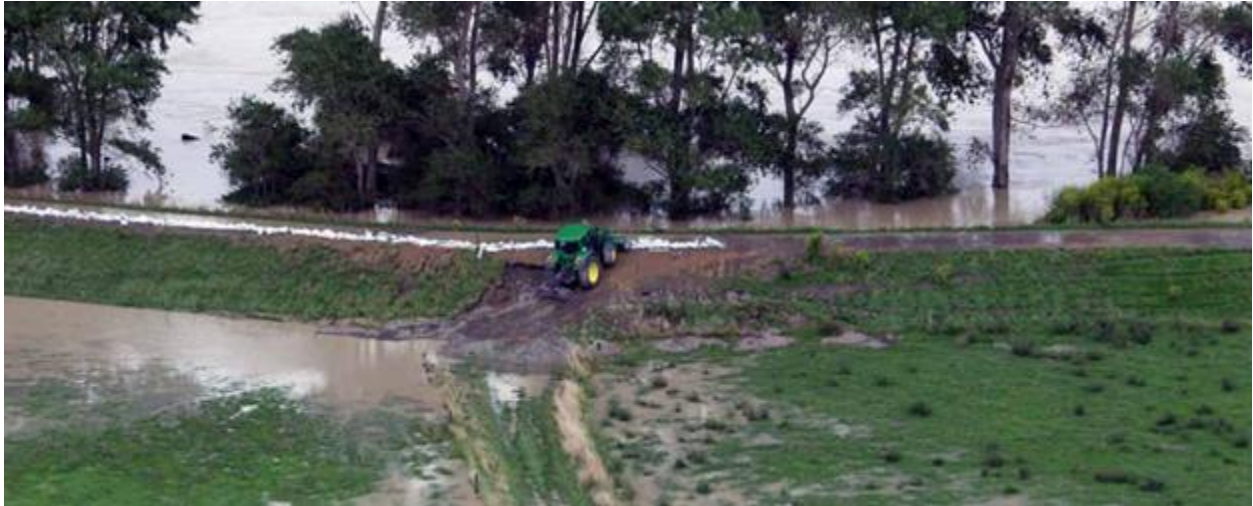
FIGURE 3: STOPBANKS ALONG THE RUAMAHANGA RIVER, [PHOTOGRAPH GWRC, N.D.]
