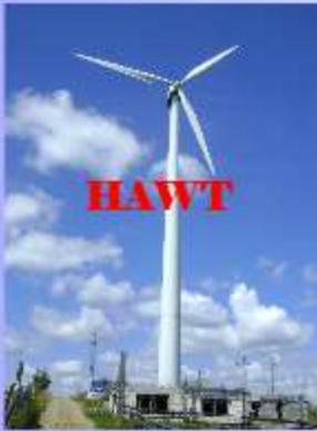
Horizontal Axis Wind Turbine
