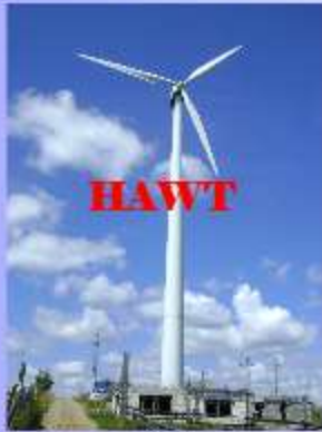
Horizontal Axis Wind Turbine
