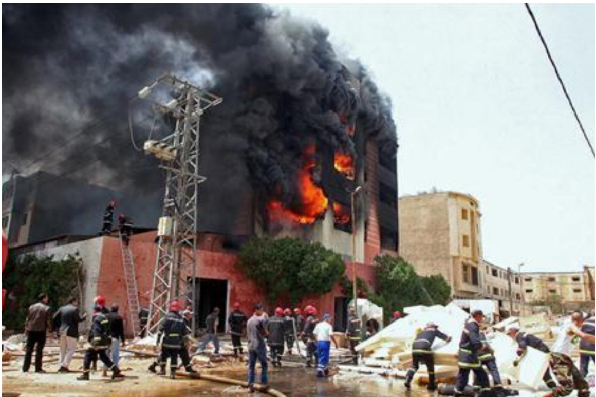
Figure 2: Fire at Mattress Factory in Casablanca (Reuters, 2008)
