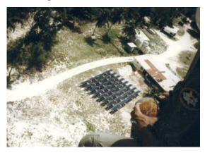
Figure 2.7: 15 kW Photovoltaic System on Mona Island, Puerto Rico (Bing, 1998)
