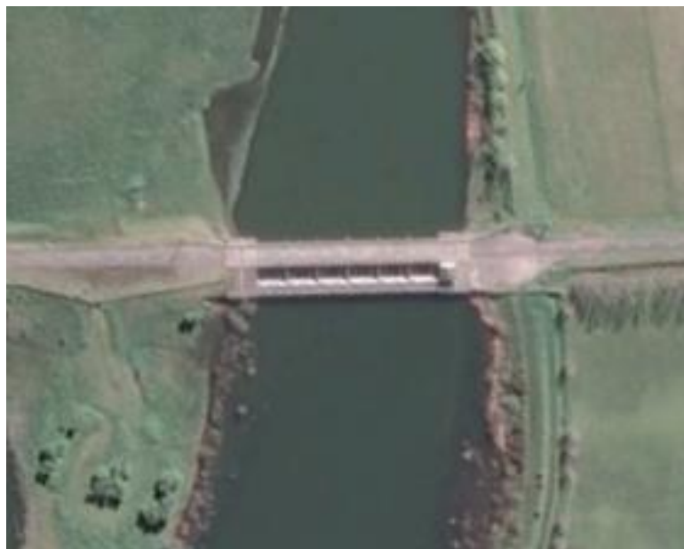
Figure 8: The Blundell Barrage gates (Google, 2015)
