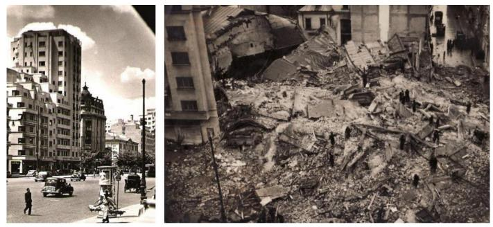
Figure 2.5: Carlton Block before collapse (left) and immediately after collapse (Georgescu & Pomonis, 2012).
