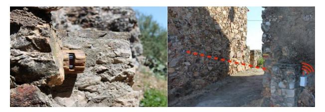
Figure 2.6: Installed Light Beam Sensor in Naturtejo National Park (Dionisio, 2016).
