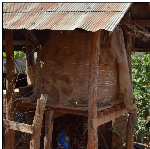
Figure 4-18: Villager Rice Storage Containers
